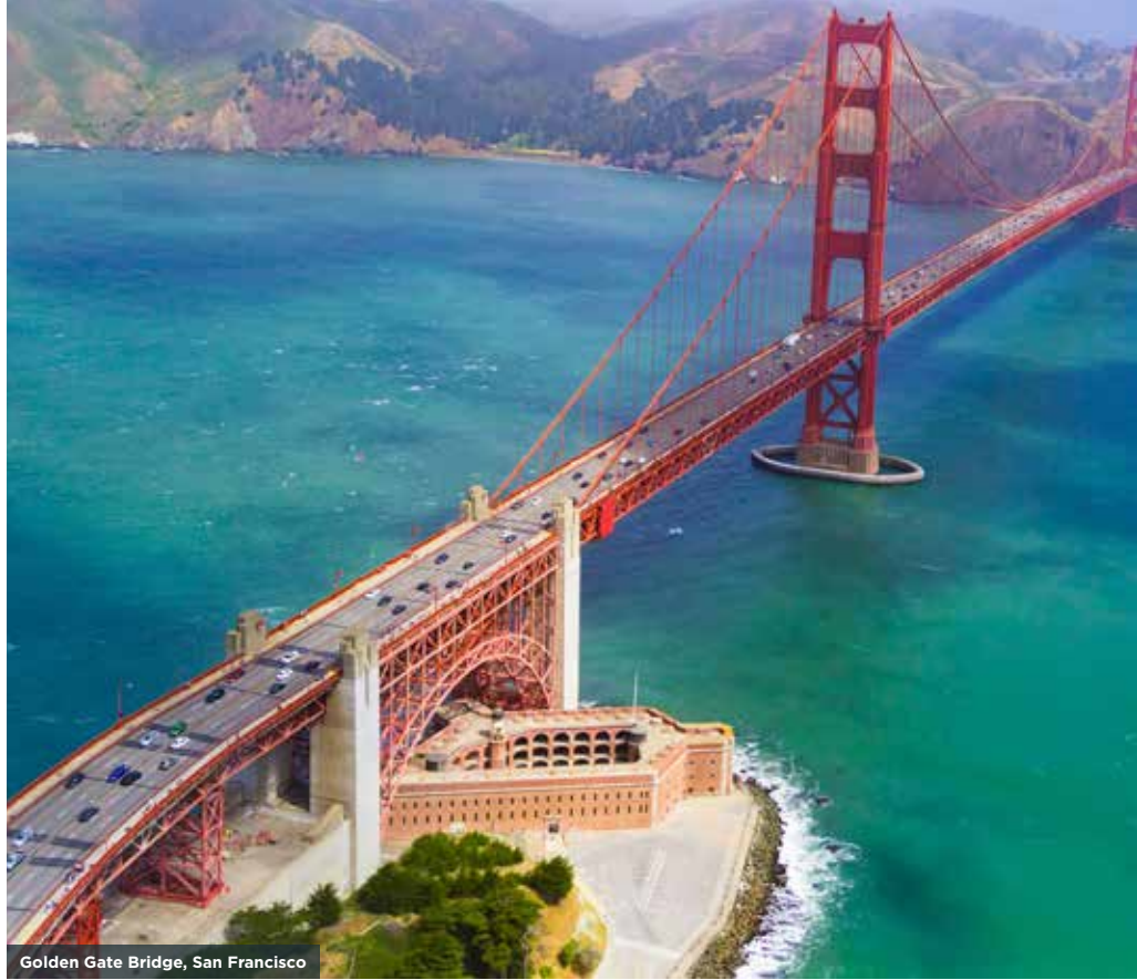
Golden Gate Bridge, San Francisco
